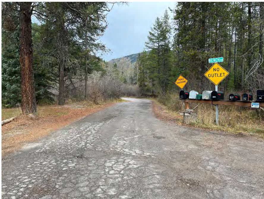
Photo #16: View of asphalt cracking and failure near Grant Creek intersection
