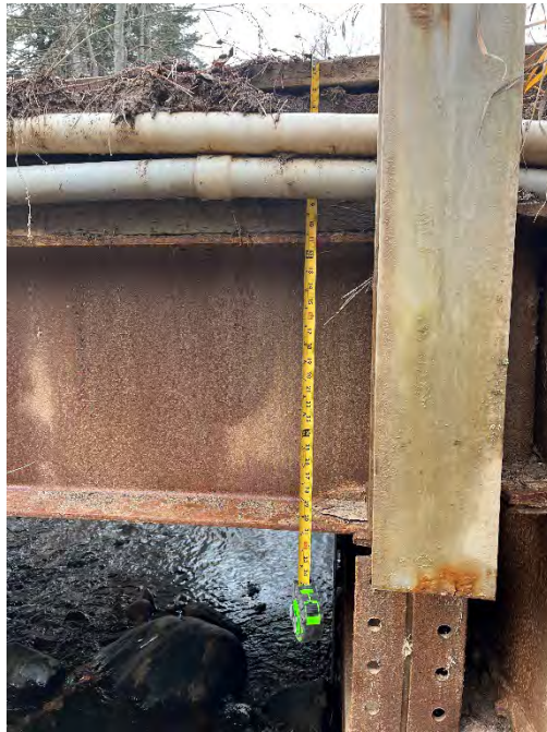
Photo #13 – View of upstream utility conduits
