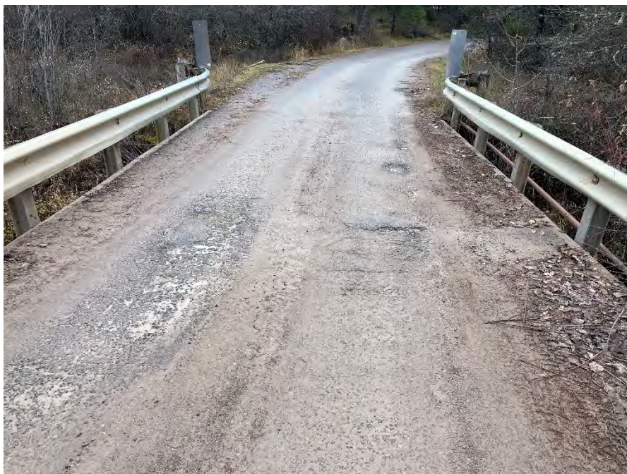
Photo #12: View of deck condition with previous asphalt loss.
