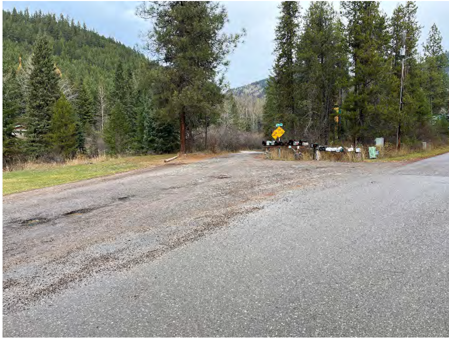
Photo #15 – View of poor quality asphalt condition at Grant Creek Road
