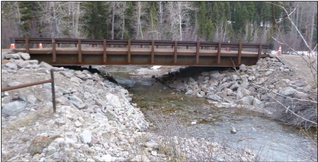
Figure 5: Example prefabricated steel girder system
