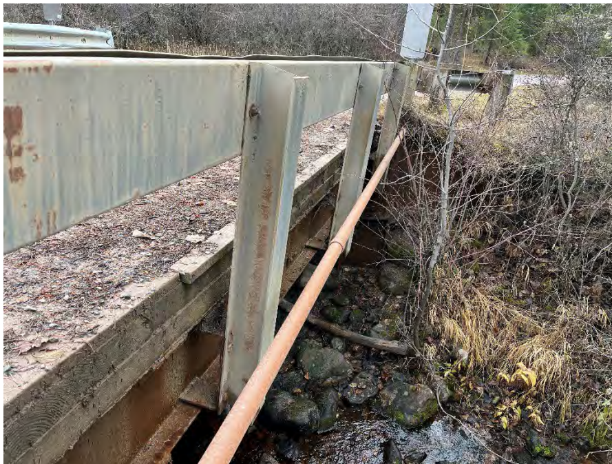
Photo #14: View of downstream utility conduit
