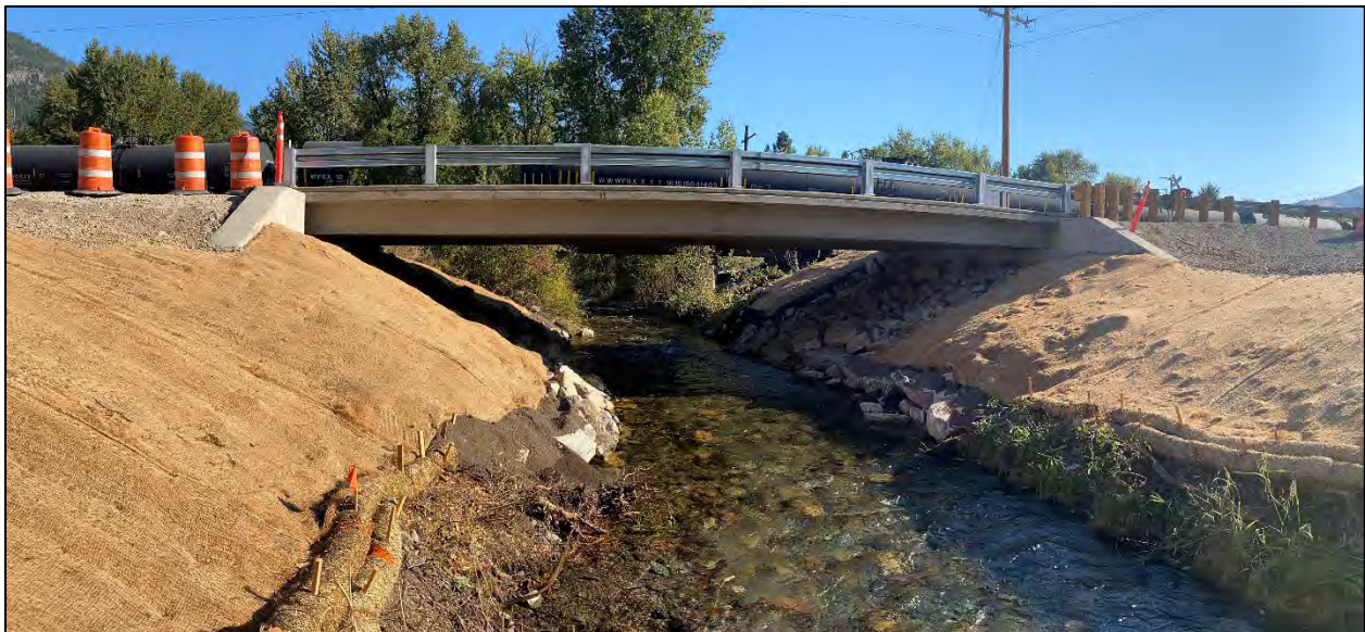
Figure 4: Example prestressed concrete girder system
