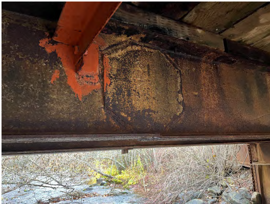
Photo #10: View of poor quality spliced girder members
