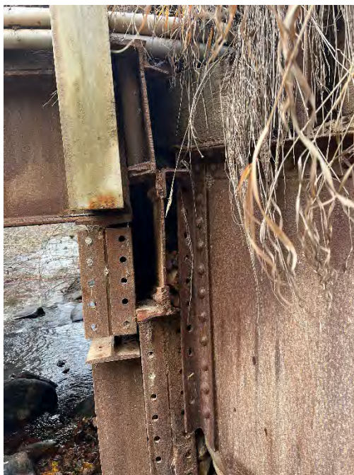
Photo #11 – View of Abutment 2 with member separation and rotation.
