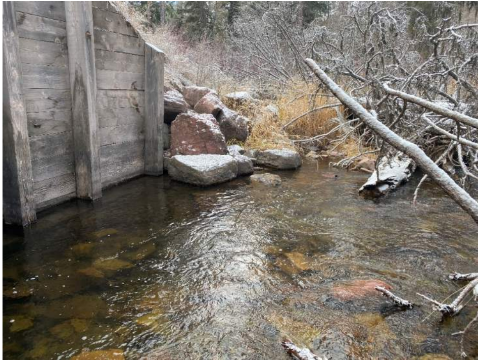
Figure 7 - Stream: Scour at Upstream Corner of Abutment 2
