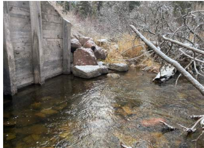
Figure 4: Upstream side of abutment 2, armored with large riprap
