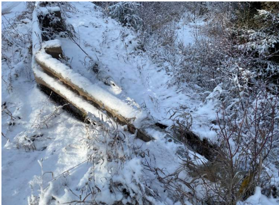
Figure 10 – Roadway Safety: NE Corner Damaged Approach Rail Terminal
