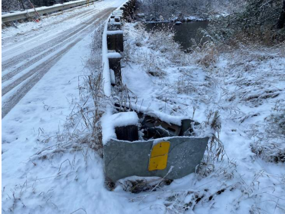
Figure 11 – Roadway Safety: SW Corner Damaged Approach Rail Terminal
