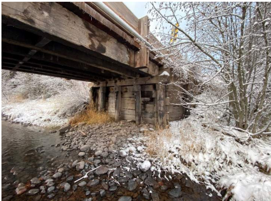
Figure 2 – Existing Bridge and Roadway: Typical Bridge Abutment
