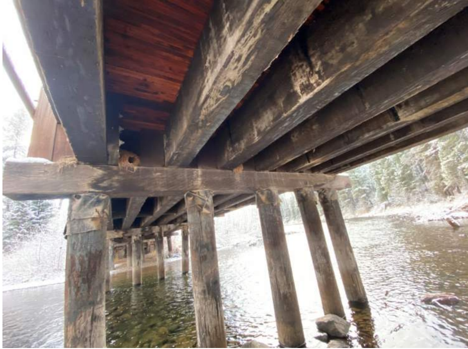
Figure 3 – Existing Bridge and Roadway: Typical Bridge Pier
