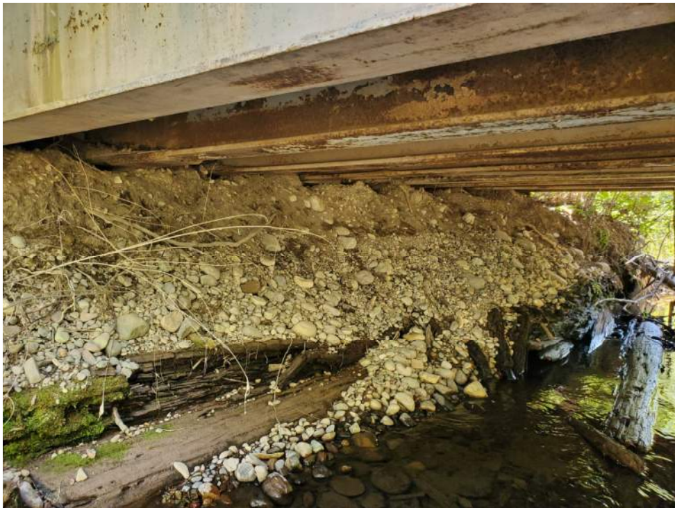
Photo 10: Example of debris build up extending above low chord at 03788.
