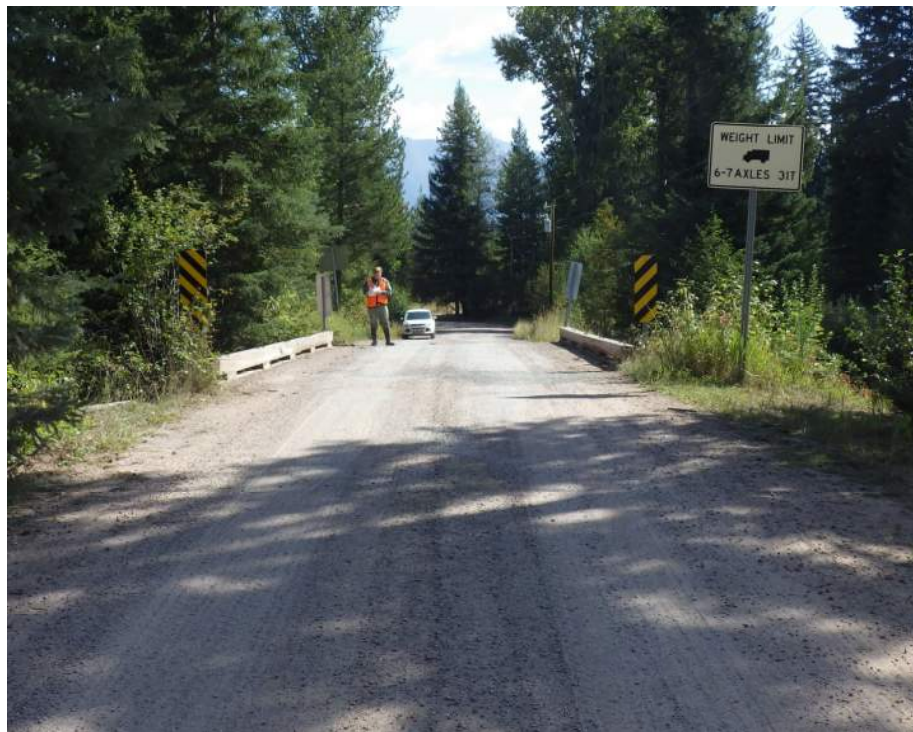
Photo 4: Top of Deck at 03787. Note substandard traffic rail, lack of approach guardrail, and load posting sign.
