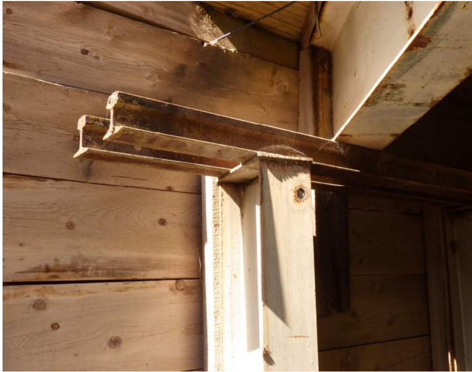
Photo 3: Non-Standard Railroad Rail Cap Beam at 03787
