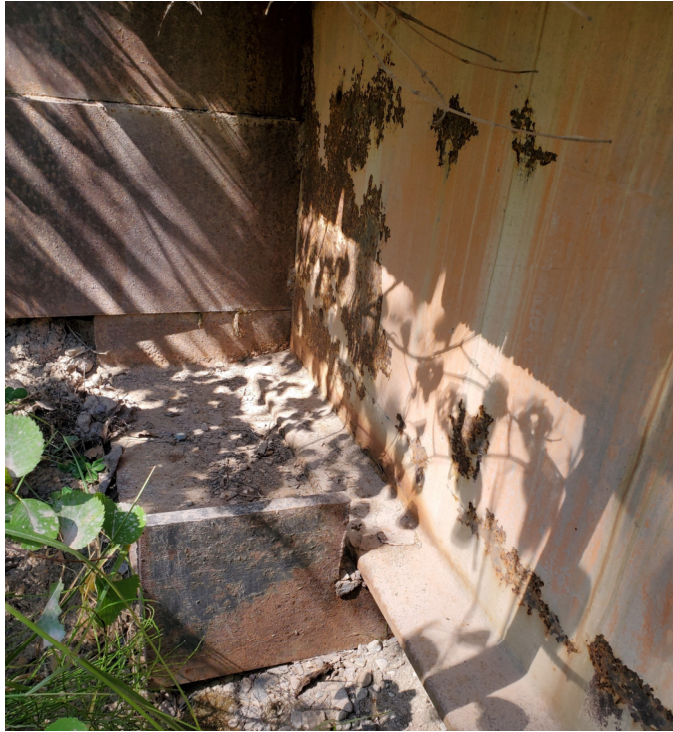
Photo 7: Abutment at 03788: Flat W Beam that support beam ends and steel plate backwall.
