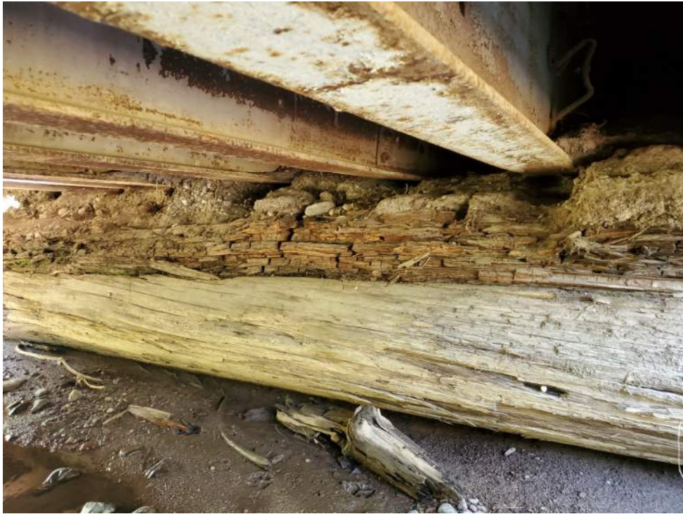
Photo 9: Example of timber logs that have been piled up in front of the bridge abutments at 03788.
