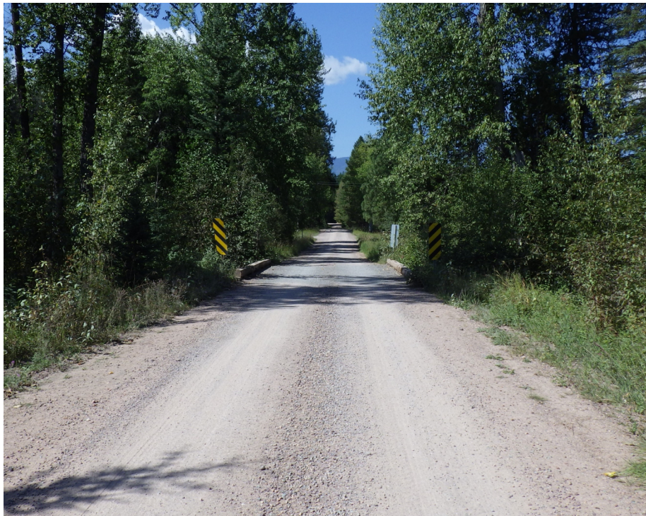
Photo 8: Top of Deck at 03788. Note substandard traffic rail and lack of approach guardrail.
