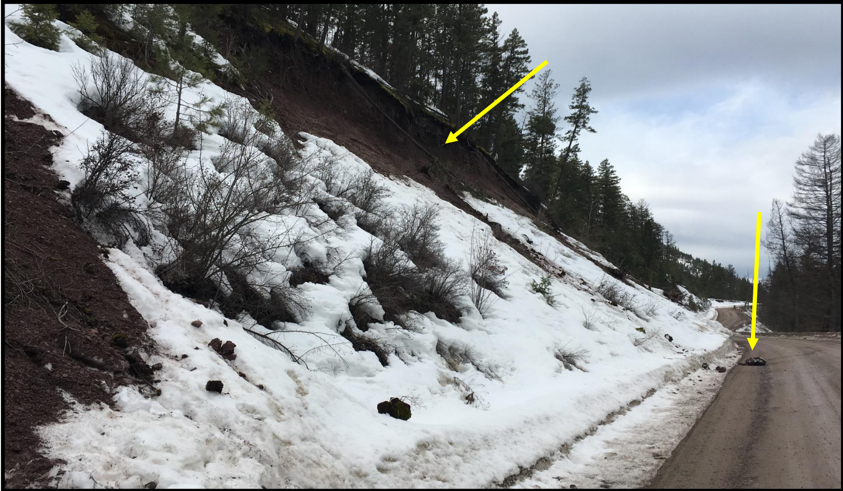
Photograph of headward slope erosion and erosional debris on Big Flat Road, Landslide Zone 7 (see yellow arrows). At this location, slope erosion progresses uphill until a sufficient overhang develops, at which time either the overhang falls off or a block of the uphill slope fails and slides downhill. Currently, such erosion primarily generally poses only a maintenance issue, but eventually, larger-scale erosion and landsliding of this slope will pose a danger to the roadway.
